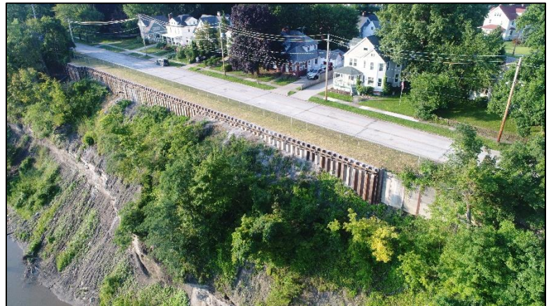
The completed shoreline stabilization project along Bank Street and the Grand River in Painesville, Ohio.
